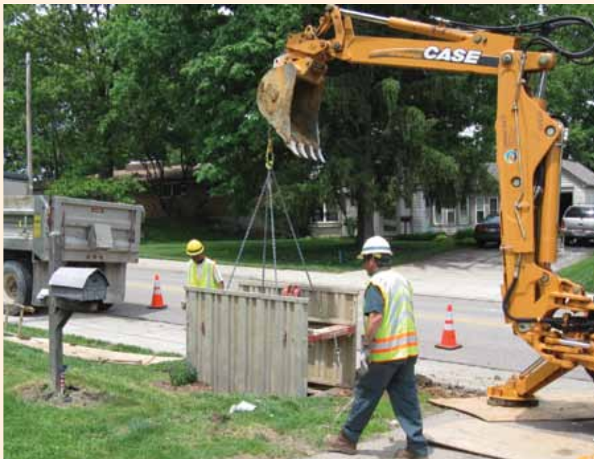
MSD personnel engaged in sewer repairs
