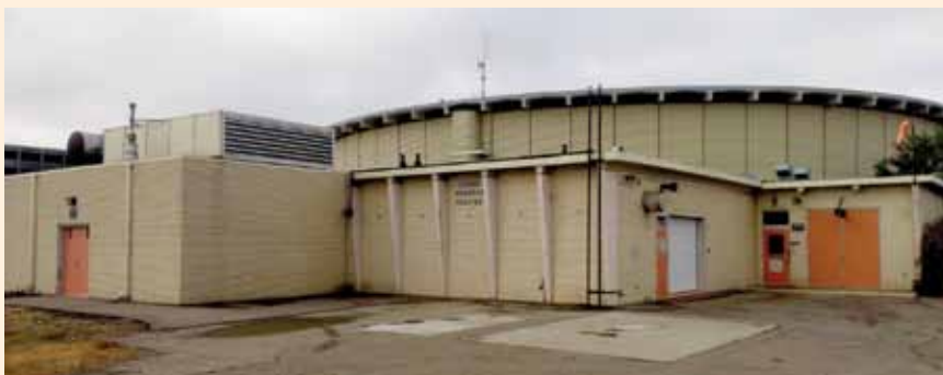
North Pumping Station
