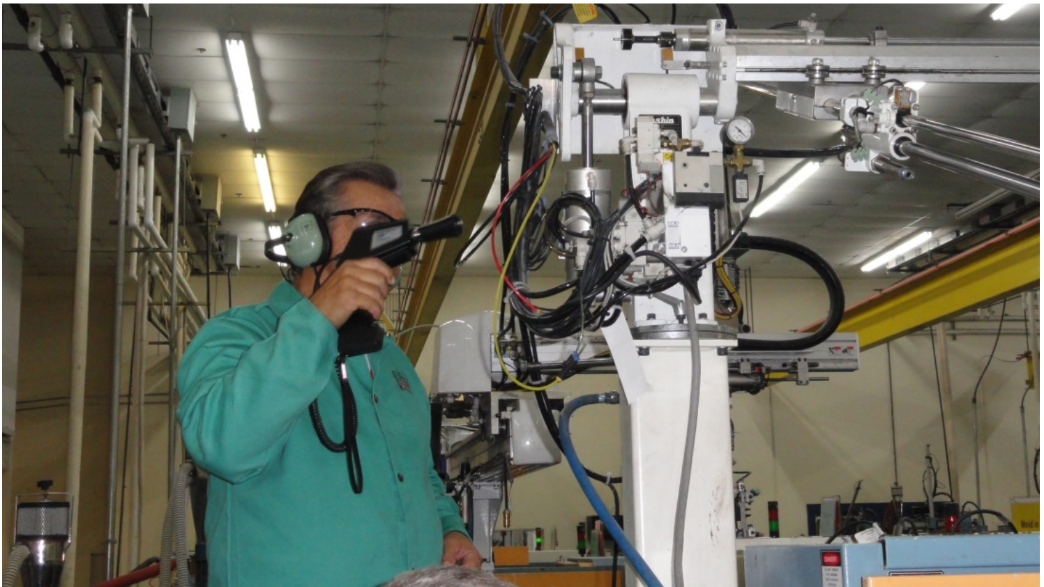
Figure 4: Technician using ultrasound to locate air leak on robotic arm. (Photo courtesy of All Leak Detection & Locate, LLC)
