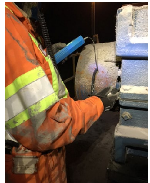
Figure 2: Operator learning to use ultrasound instrument that allows the individual to find temperature of bearing as well as datalog decibel reading, tachometer, accelerometer, as well ultrasound sensors, bluetooth and record bearing sound for further diagnostics.
