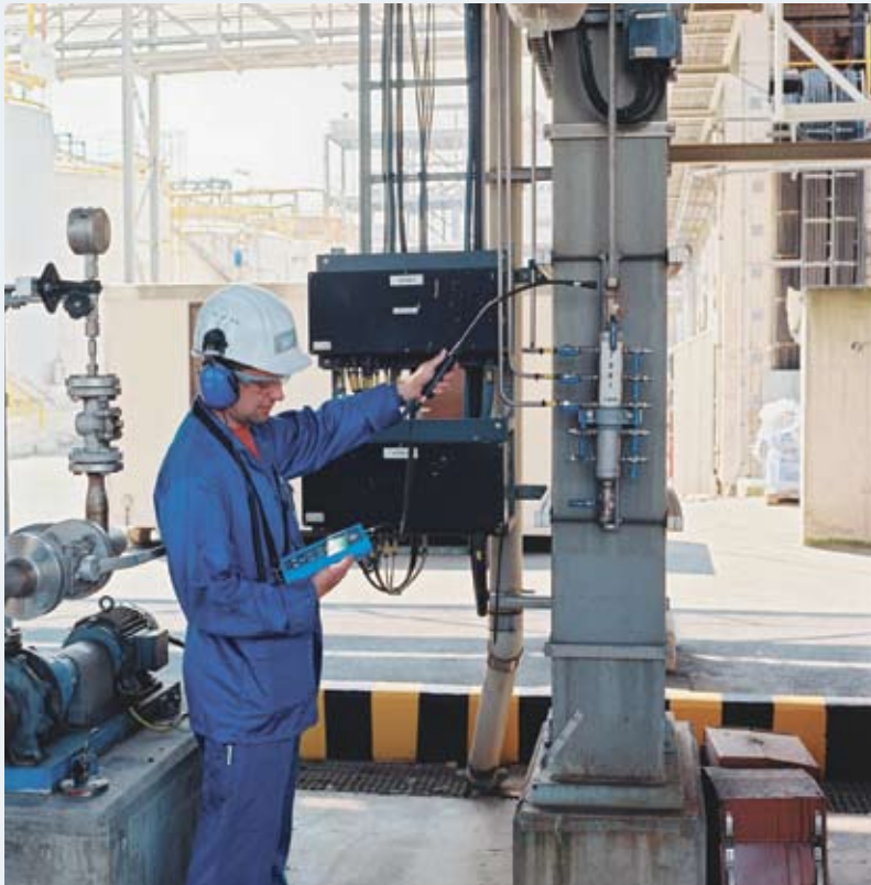
Figure 3 - Conducting an Air Leak Survey.
