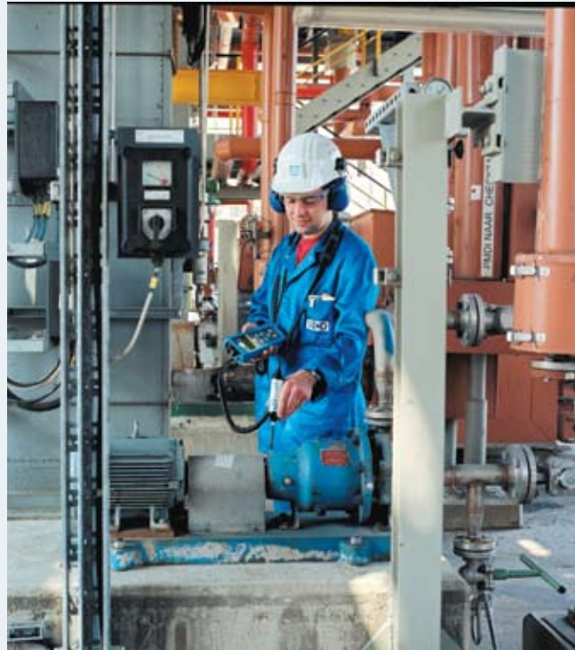
Figure 12 - Checking Cavitation
