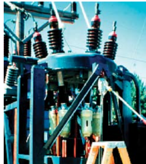
Figure 1 - A set of 3-phase oil-filled circuit breakers (OCBs) seen from the outside (left) and another set (right) from the inside, with the oil drained, showing part of the bushing structure and contacts.
